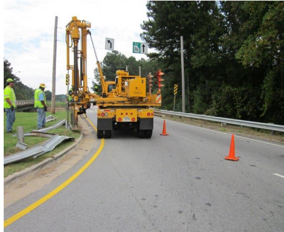
D3 Guardrail Repair
