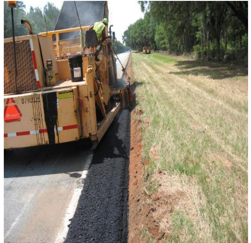
D4 2FT Shoulder Paving
