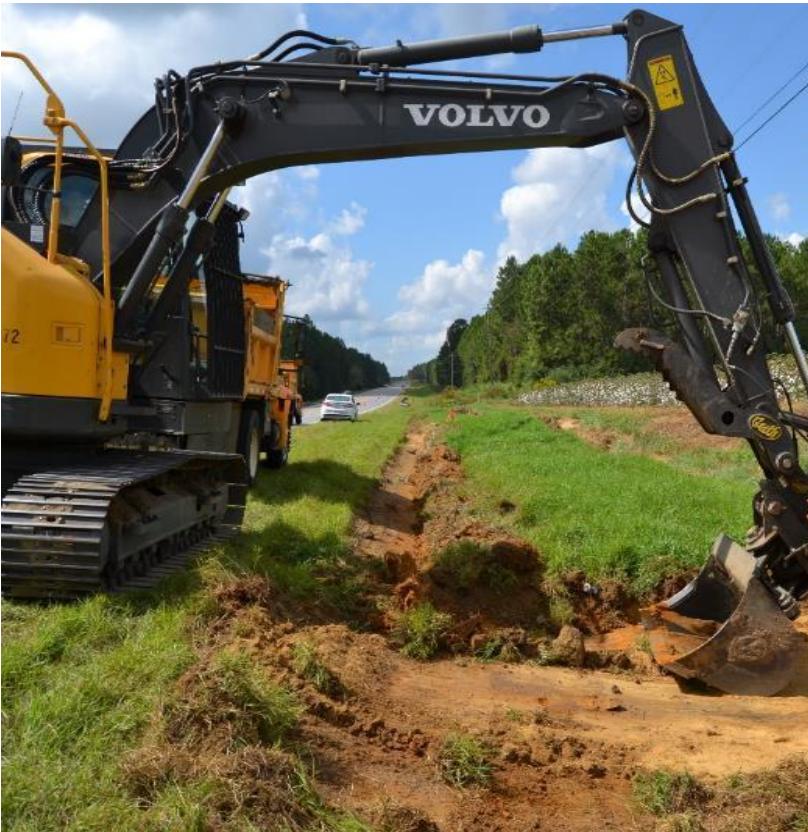
D4 Ditch Cleaning – US 319 Colquitt
